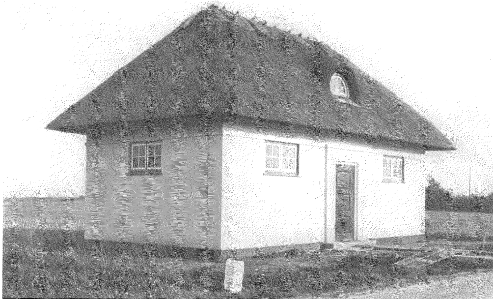
Fig. 13—Brondby Vester District Exchange—Denmark—600 Lines Capacity.
