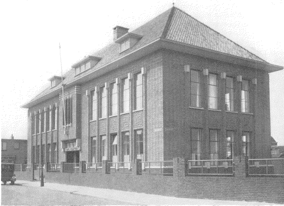
Fig. 12—Ymuiden Centre Exchange—Haarlem Rural Area—Holland—4,000 Lines Capacity.
